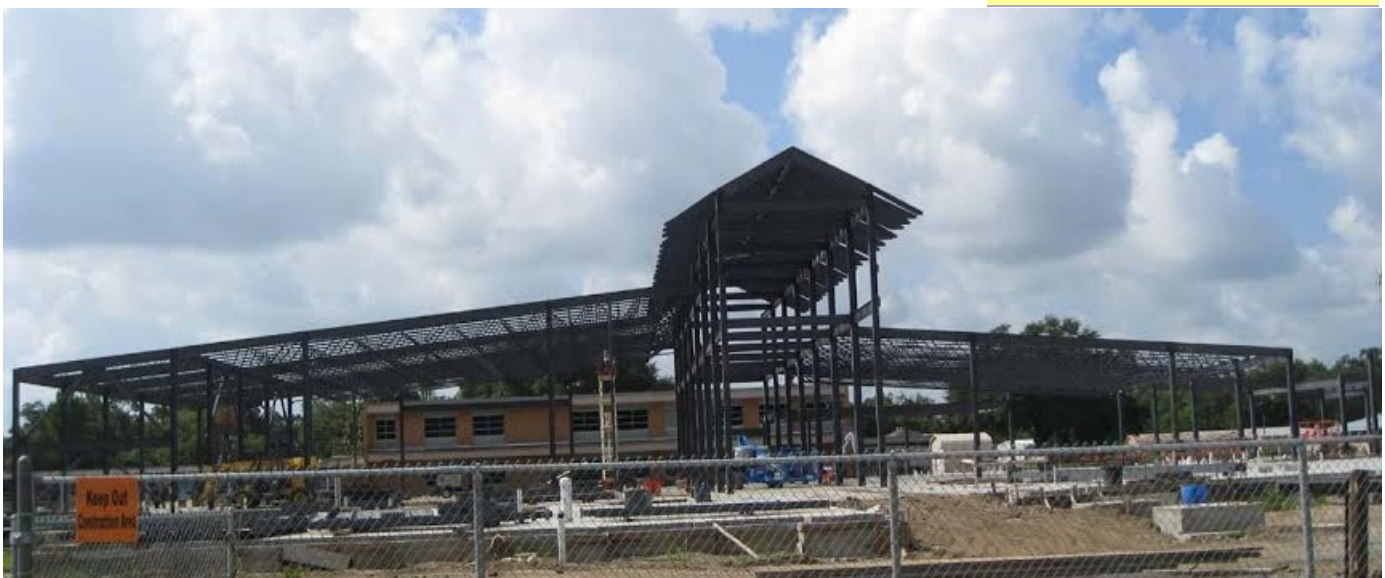
New On-going Patterson Jr. High School Structure—Work In Progress
